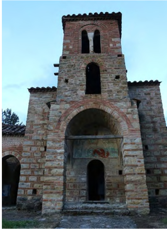
Ill. 131. The tower in front of the narthex of the church of St. George in Omorfoklisia (between 1295 and 1317). Photo: S.V. Maltseva
