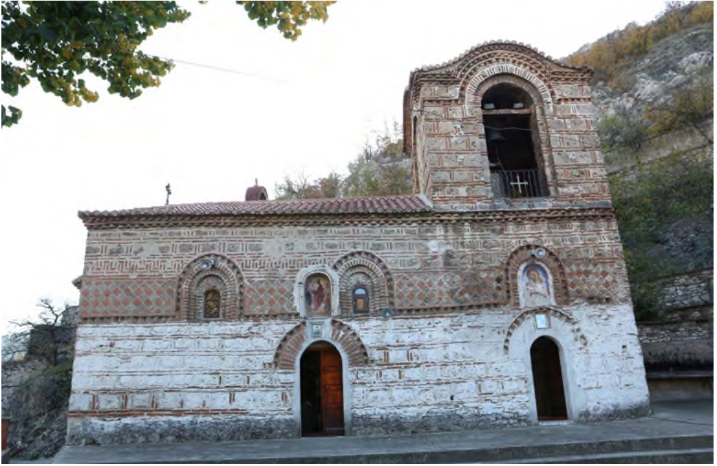
III. 110. Church of St. Demetrius in Veles, northern facade (1297). Photo: S.V. Maltseva
