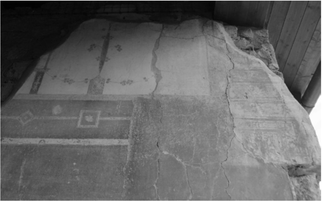
Fig. 5. The cut in the Third Style wall decoration of the NE wall of vestibulum 46 and in the center the poor quality plaster patch © Parco Archeologico di Pompei
