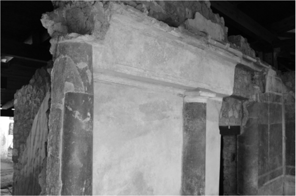
Fig. 4. The cuts and the red stucco reconstructions visible on the false porticoed structure in room 86 © Parco Archeologico di Pompei
