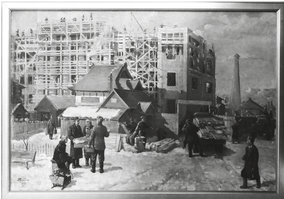
Fig. 2. Pavel Pogodin. Construction Site of Fishery Office. 1950. Sakhalin Regional Art Museum, Yuzhno-Sakhalinsk
