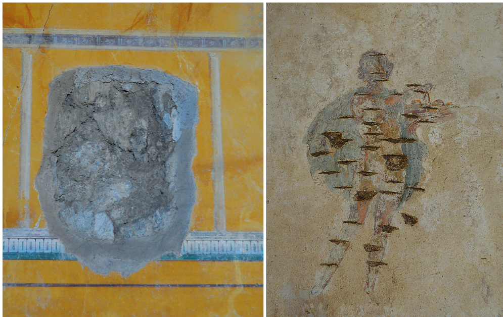
Ill. 97. On the left, the void in the wall left by the 18th century excavators after stripping off the painting; on the right, intentional destruction of the wall decoration, Villa Arianna, Stabiae. With the permission of the Ministero dei Beni e delle Attività Culturali e del Turismo — Soprintendenza Pompei. All rights are reserved.
