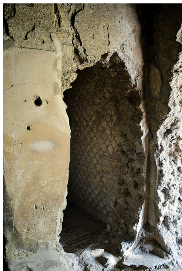
Ill. 101. Breach made by the excavators in the wall between rooms 26 and 27 in Villa San Marco, Stabiae. With the permission of the Ministero dei Beni e delle Attività Culturali e del Turismo — Soprintendenza Pompei. All rights are reserved.
