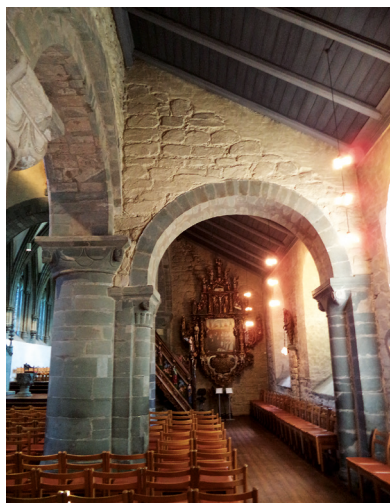
Ill. 78. Diaphragm arch in the south aisle of St. Swithun cathedral in Stavanger. Photo by K. Chemezova, 2013.
