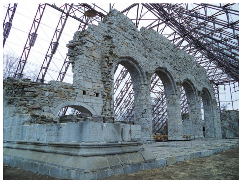
Ill. 77. Southern arcade of Christ cathedral in Hamar. Photo by K. Chemezova, 2013.
